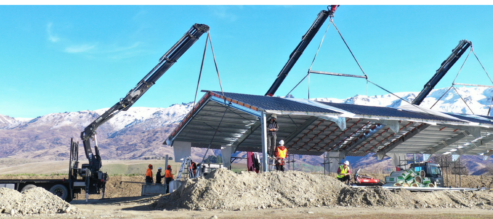
H ROOFING & CLADDING
