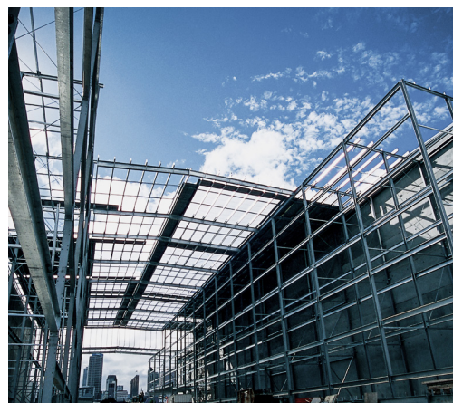
(B) STRUCTURAL STEEL, HST PURLINS & GIRTS
