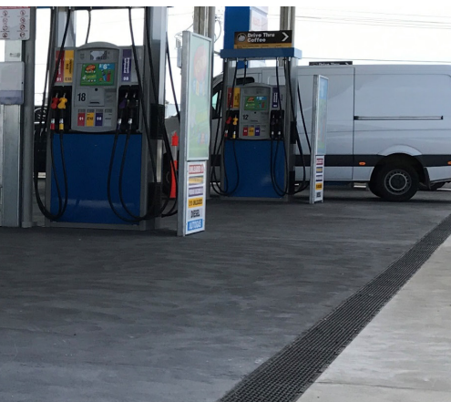
C ORCA POLYMER CONCRETE CHANNELS
