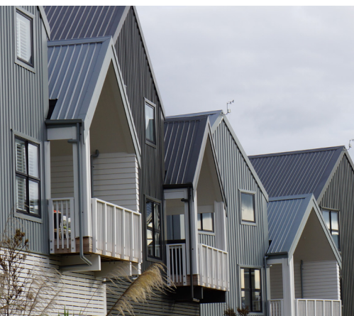
(A) METAL PROFILE ROOFING & CLADDING
