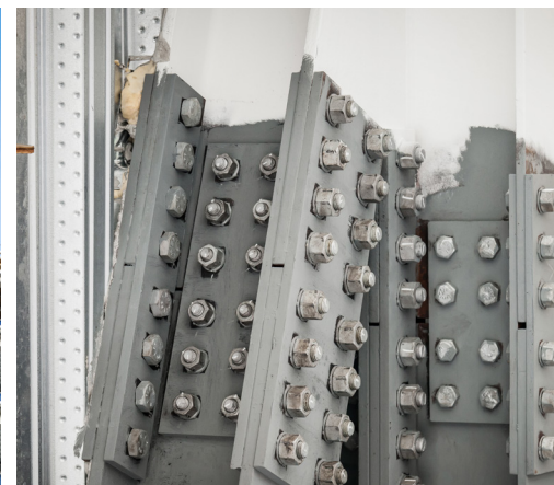
(F) PRE-DRILLED PLATE & STRUCTURAL BOLTS
