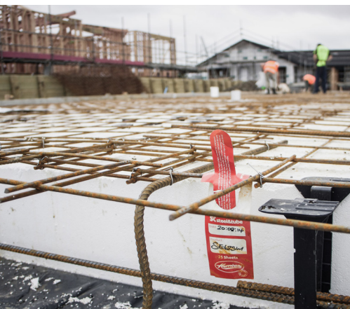
(C) RESIDENTIAL FLOOR MESH & SLAB REINFORCEMENT
